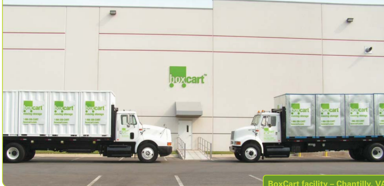
BoxCart facility – Chantilly, VA
